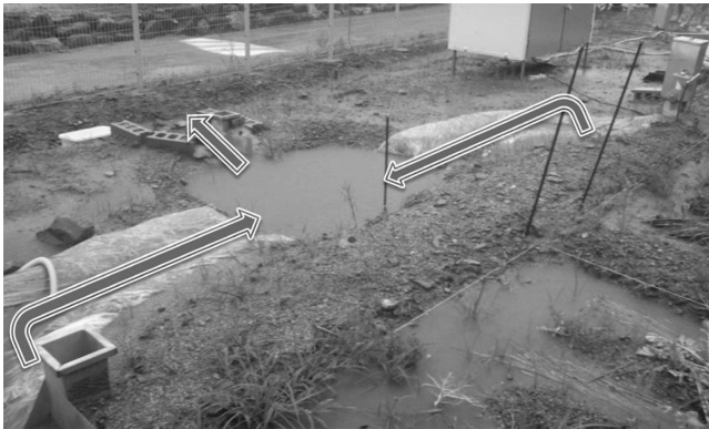
Fig. 2 Route of inlet and outlet discharge at sediment trap
